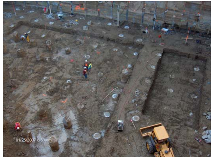
Fig. 8. Trimmed LCCs and reinforced foundation subgrade
