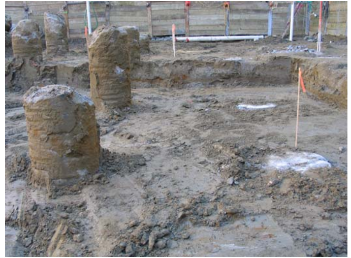
Fig. 7. Tops of LCCs before and after trimming
