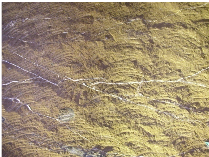
Fig 15. SILACSOL permeation through the cracks system as appeared during the tunnel excavation
