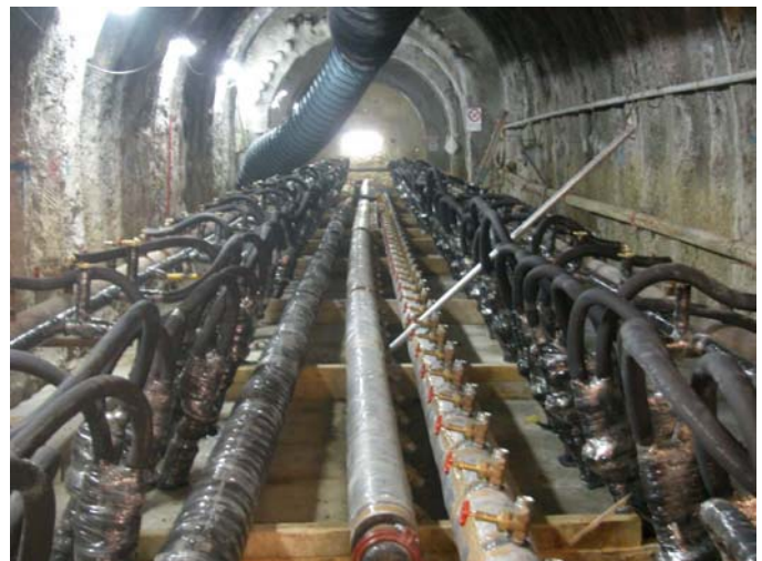
Fig. 23. Drift manifold system and inclined freeze-lances
