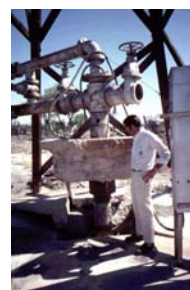
Fig. 1: Water well installation seems to rise in the air due to land subsidence
