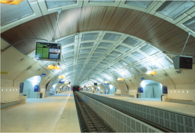
Fig. 3: Completed central tunnel
