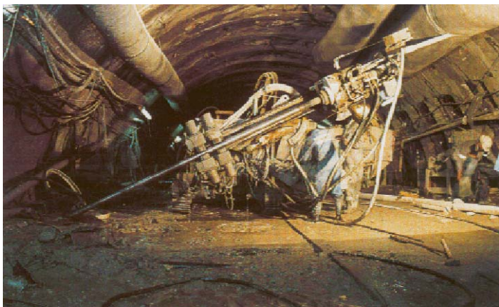
Fig. 8: Jet grouting from inside tunnels
