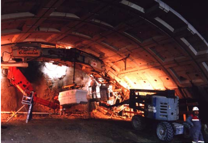
Figure 9: Construction of the active vault
