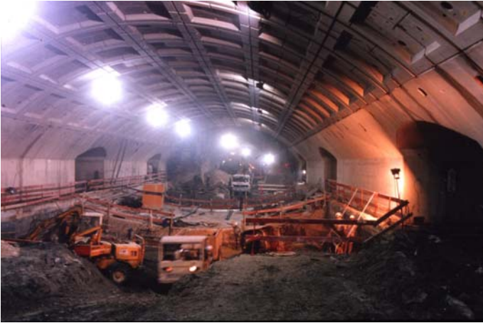
Figure 10: Completed active vault
