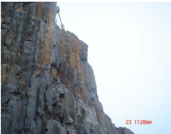
Fig. 2. View of columnar joints
