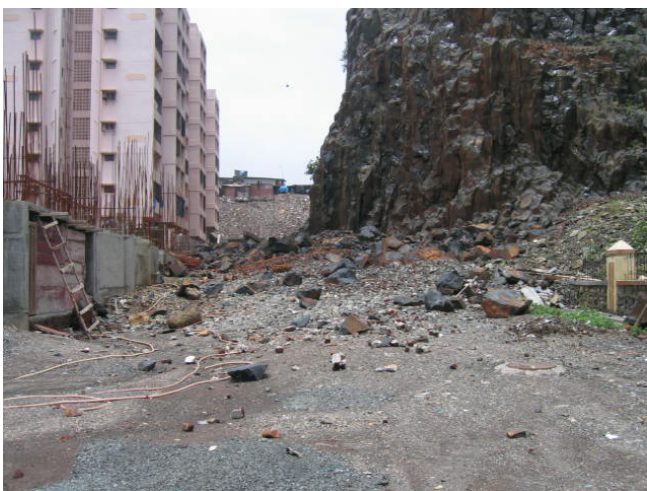
Fig. 4. Debris after heavy rain fall
