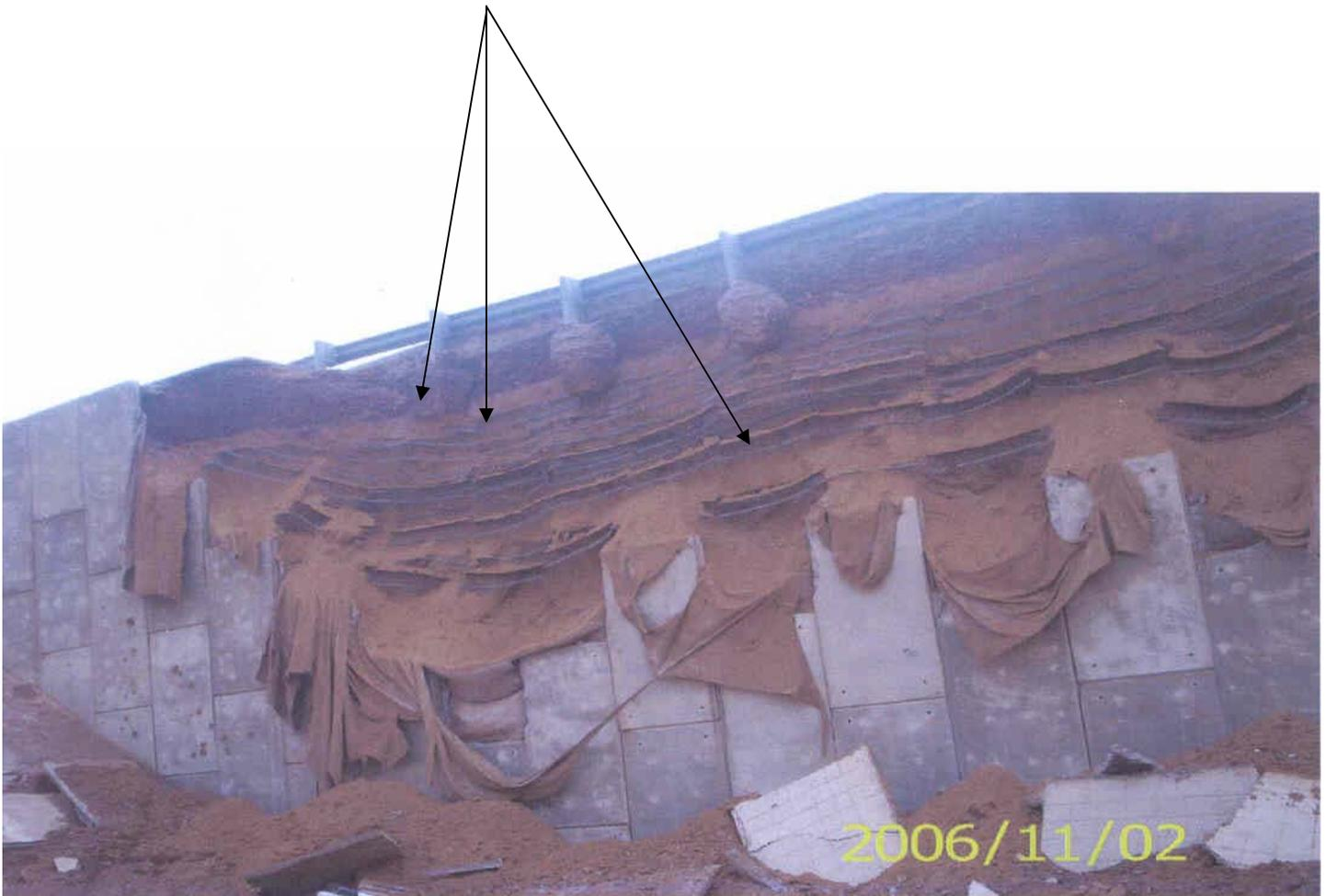
*Fig.3.View of collapsed RSR wall, Exposed Geogrids are seen over the collapsed fill*
