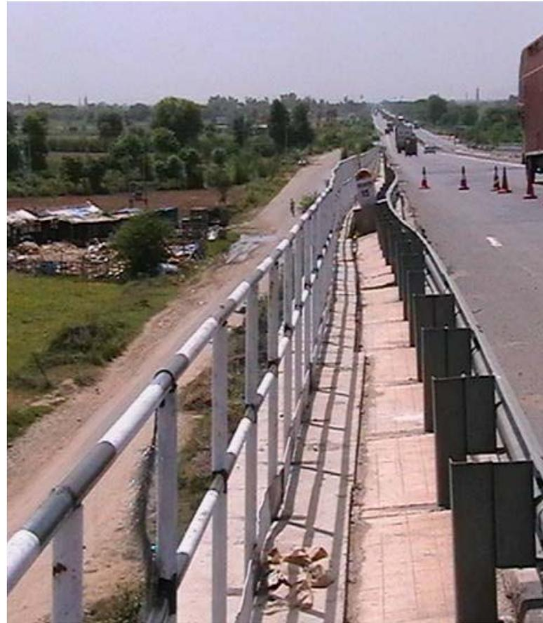
Fig. 2: Guard rail and pipe moved out of alignment due to large outward movements of Facia Panels
