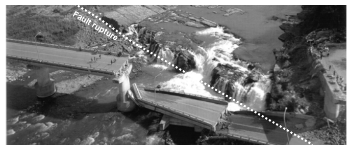
Fig. 1. Collapse of two spans of the Bei-Fung bridge due to tectonic dislocation in the 1999 Chi-Chi (Taiwan) earthquake.
