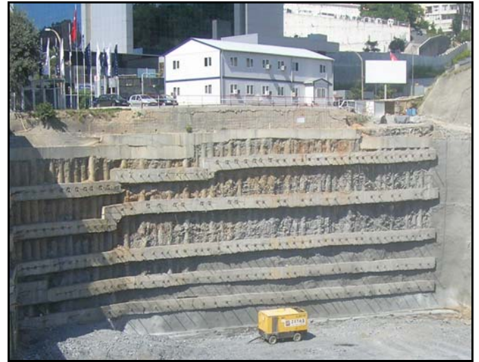
Fig. 12d. Reinforced concrete walls under the bored piles
