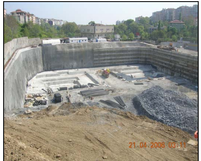
Fig.13a. Retaining system facing north side
