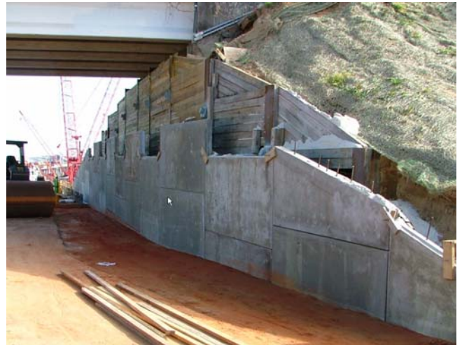
Photo 4: Panel Wall Construction
