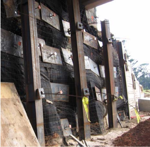
Photo 3: Soldier Pile Wall with Tieback Anchors
