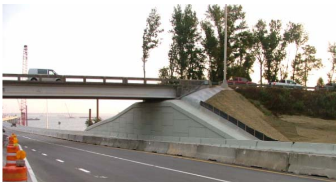
Photo 5: Final Finished Wall
