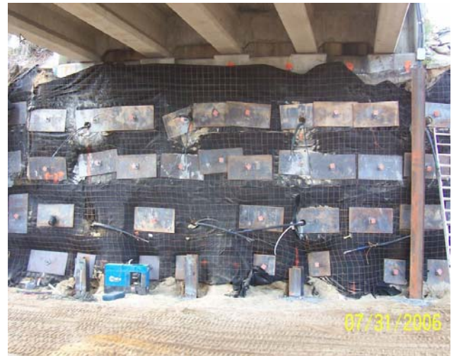
Photo 2: Flexible Facing of Temporary Excavation Support
