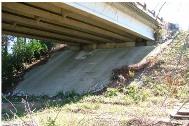
Photo 1: South Abutment of Scenic Highway
