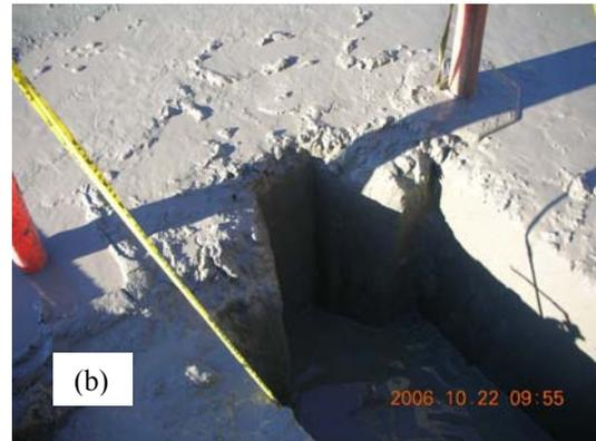
Figure 11 – (a) Installation of CWS End Joint Forms; (b) Key Slot formed by CWS End Joint System
