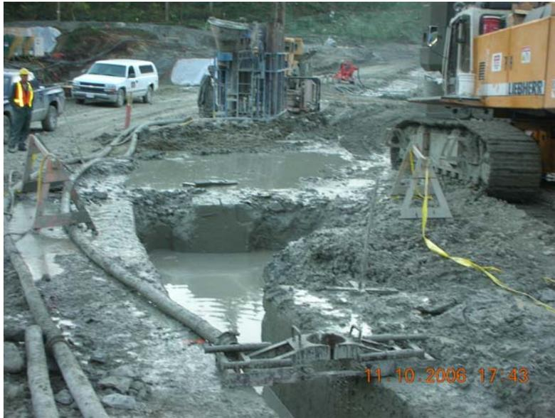
Figure 12 – Cross Bite Excavation at Panel Joint Location to remove boulder and CWS End Joint Forms
