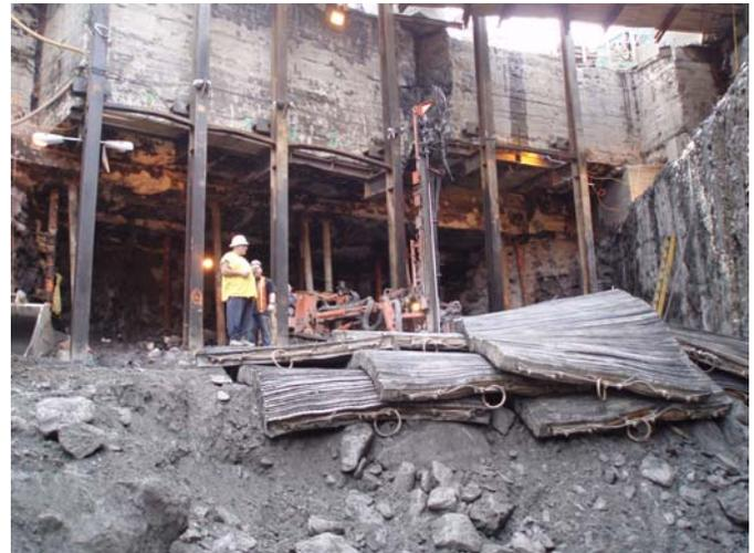
*Fig. 3. Blasting beneath subway, between underpinning piles*
