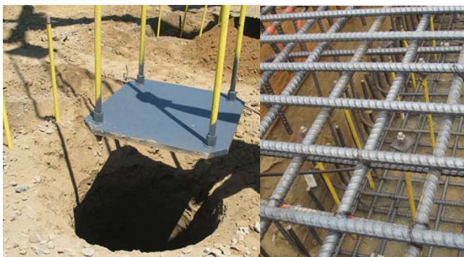
Fig. 1 RAP Uplift Bottom Assembly and Top Anchor
