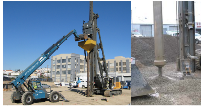
Fig. 2: Impact pier equipment with standard rammer head
