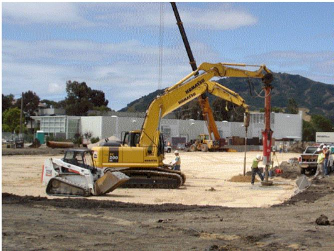
Fig. 2. Typical RAP installation equipment.
