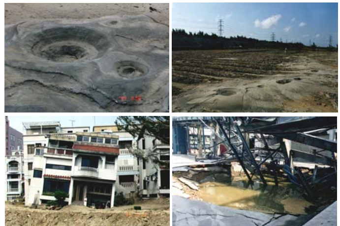
Fig. 1. Liquefaction phenomenon and induced damage in 1999 Chi-Chi earthquake
