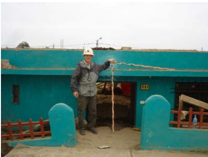
Fig. 6. Approximately 0.9 m of liquefaction-induced settlement at a one-story house in Tambo de Mora.
