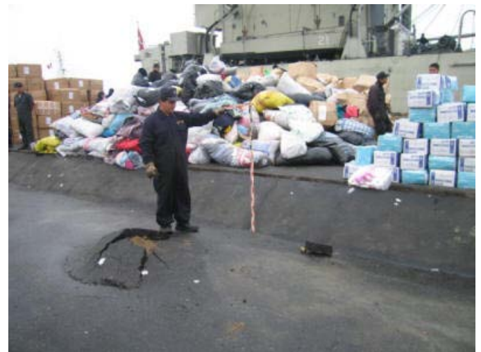
Fig. 7. Vertical displacements as large as 0.8 m were observed between the pile-supported wharf and the reclaimed
