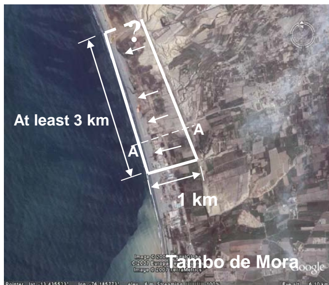
Fig. 8. Approximate extent of a massive seaward lateral spread of a marine terrace in Canchamaná. The boundary of the mobilized area on the north is uncertain and could possibly extend further (Background image from Google Earth).
