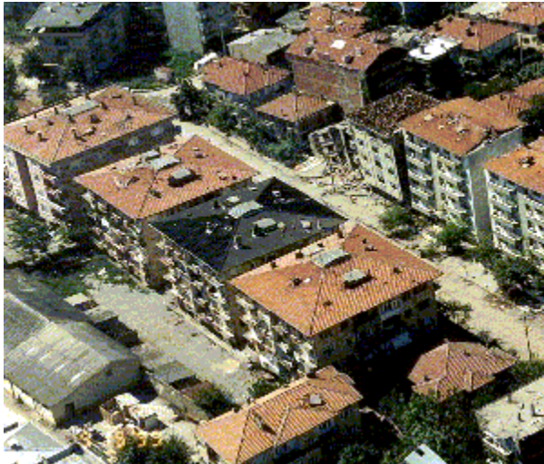
Fig. 3. Structures located at the corners (photos from peer.berkeley.edu)
