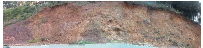
Fig. 12. View of a slope cut
