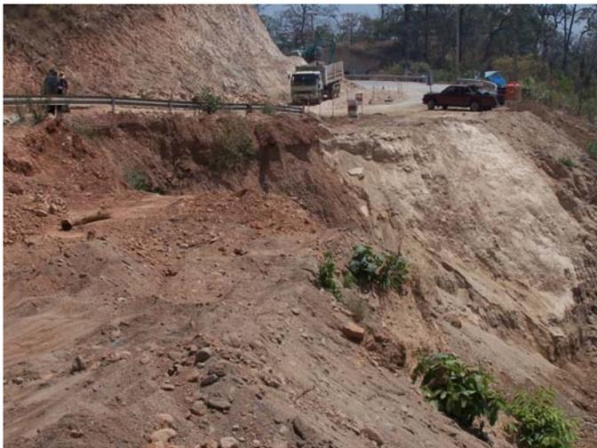
**Figure 2:** Site with Sloped Embankment Failure
