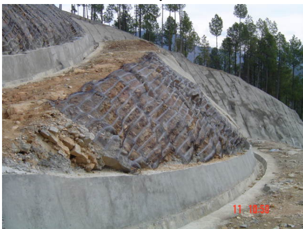
Fig.7-Slope stabilisation measures & construction of side drain on the benches in Crown Area
