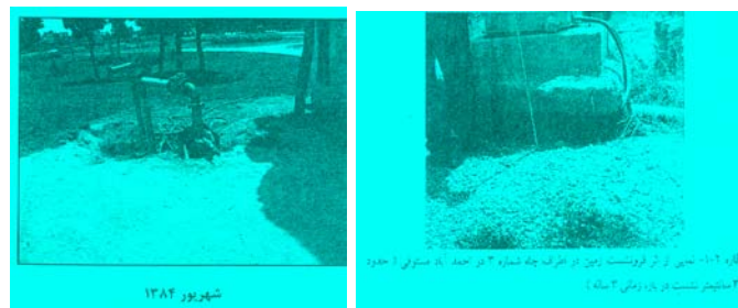
Figure 1: Water well installations seems to rise in the air due to sediment's compaction
