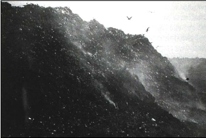
Fig. 3. Front slope of the MSW before slope failure showing surface fires and steep slope of the MSW (Kocasoy and Curi 1995).
