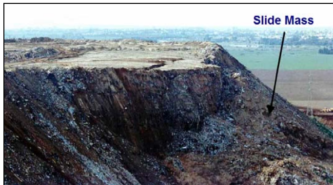
Fig. 6. 1997 Hiriya landfill slope failure (Isenberg, 2003)
