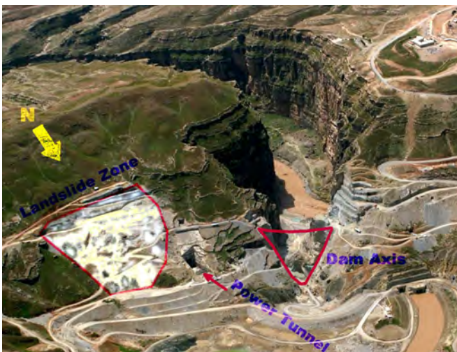
Fig. 1. Situation of landslide zone adjacent to the power tunnel entrance
