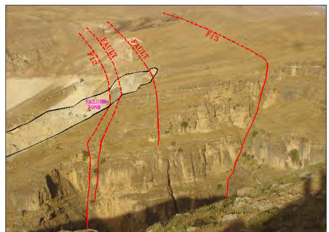
Fig. 7. The extension of tension faults and major joints in the left bank (view from the west)
