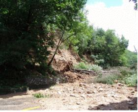
Fig 5. Schematic of slope failure due to surface runoff Fig 6. Picture of slope failure due to surface runoff
