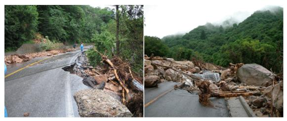
Fig 17. Loss of road by the boulder flow
