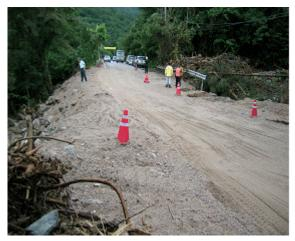
Fig 14. Damage to a road due to overflowing water
