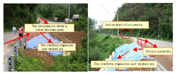
Fig 10. The damage example due to washing of fill material
