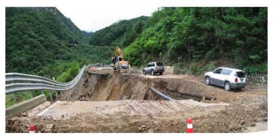
Fig 9. The damage example by banking section
