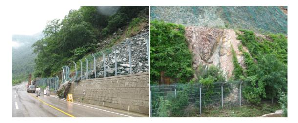
Fig 4. The Damage Example due to Stone falling
