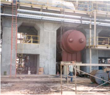
Fig. 10. View of restored STG structure.
