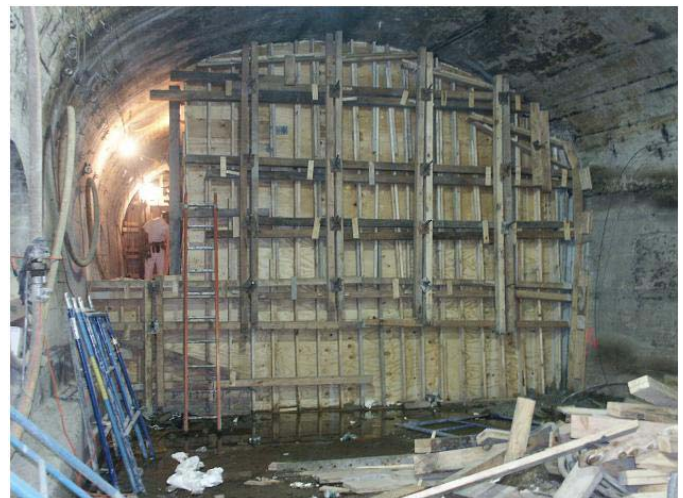
Fig.10 Formwork for Tunnel Backfilling
