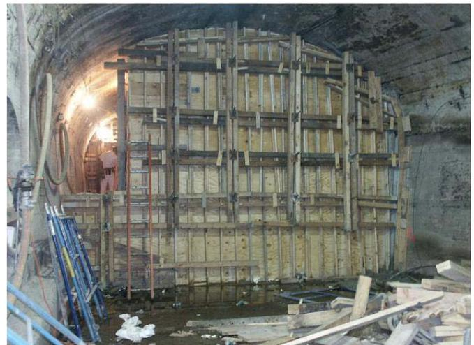
Fig.10 Formwork for Tunnel Backfilling
