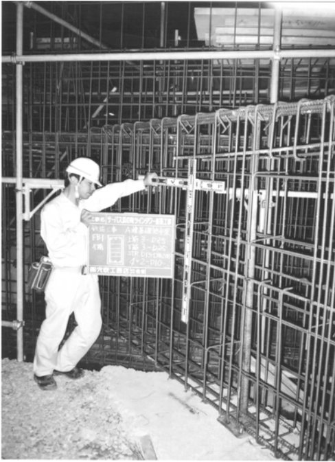
Fig. 32. Large grade beam for 14 storey building.
