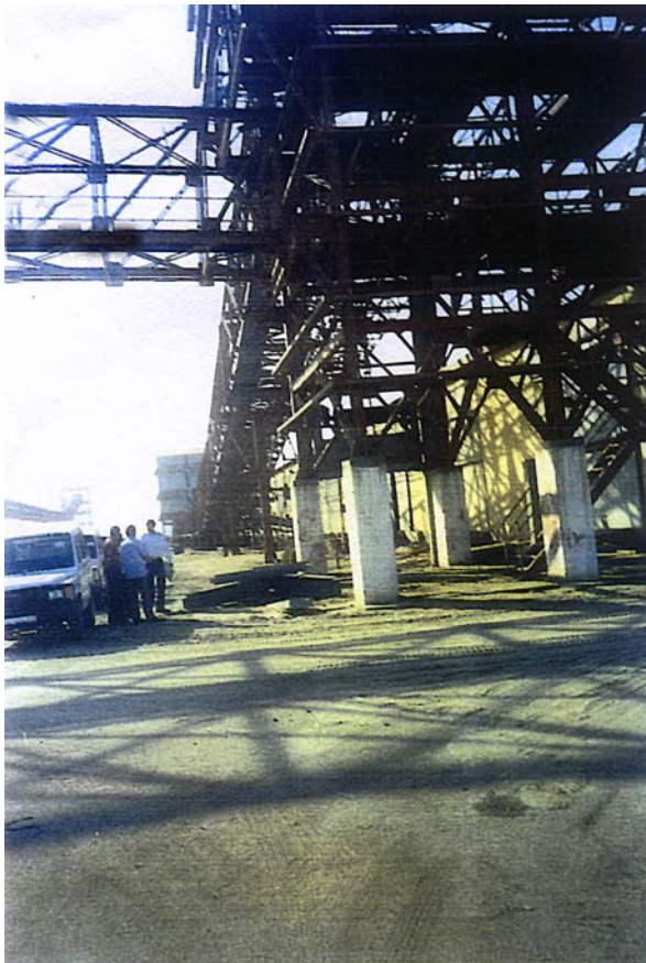
Fig. 2. Bund area parallel to the conveyer belt
