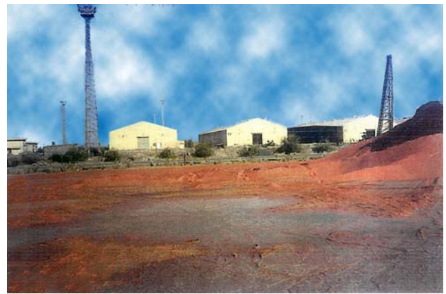
Fig. 3. Open stacking yard and dry cargo area
