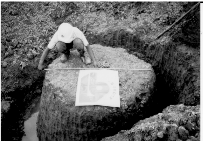
Fig. 7. Jet grouted piles after installation.
