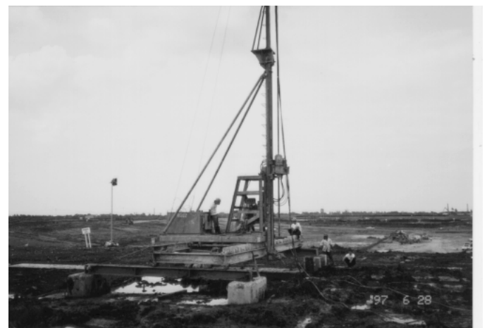
Fig. 5. Jet grouting method in construction site.
