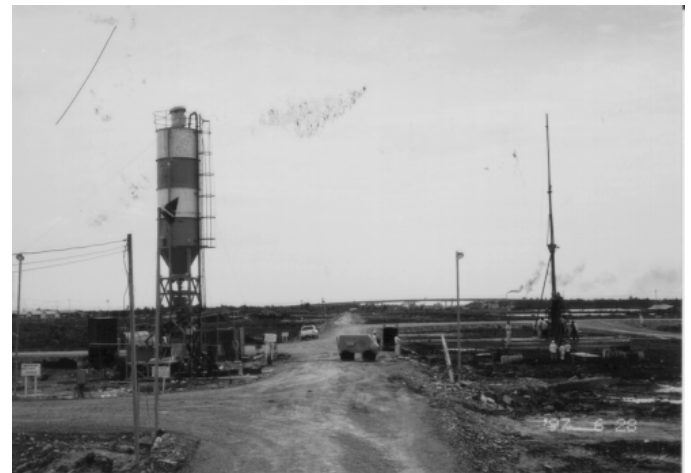
Fig. 4. Jet grouted installation at the site.
