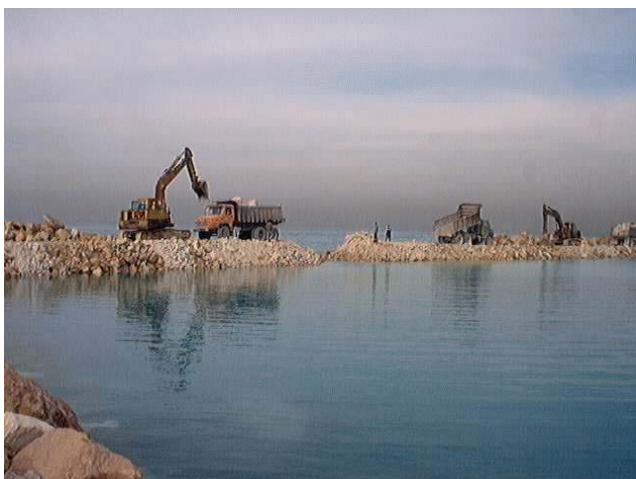
Fig. 2. A view of basin construction
