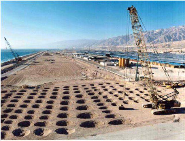
Fig. 5. A view of dynamic compaction in Assalouyeh
