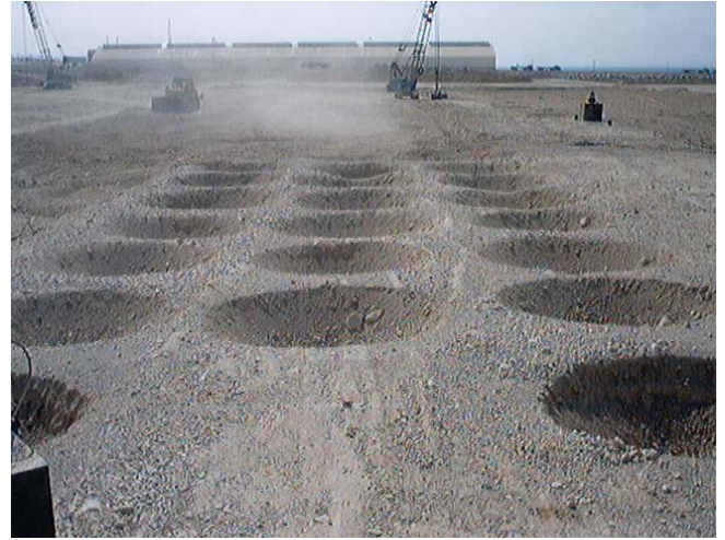
Fig. 6. Craters induced up to 2m formed at the impact points
