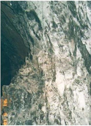
Fig. 3. Side wall scaling in 1571m cross-cut drift
