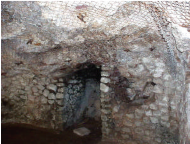
Picture 1. Masonry in a main chamber wall.
