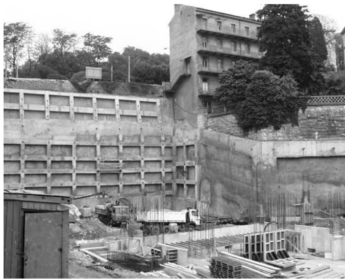
Fig. 2. Cut "North" and "East", in an excavation phase of the bottom of the open pit
