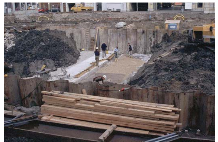
Fig. 5. Excavation and placement of the bottom slab in slices.
