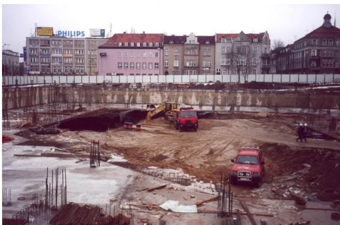
Fig. 5. General overview of excavation at “-1” level stage. The “-1” parts of permanent floor slabs (the rest of floor has been carried out in further phase of works).
