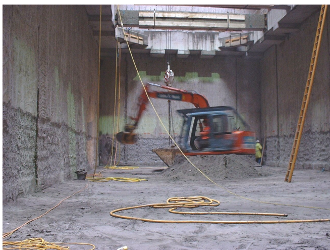
Fig. 4. & 5. Photographs taken during the 47m deep internal excavation of the shaft showing the shaft viewed from the surface and the diaphragm walls just above the maximum excavation depth.
