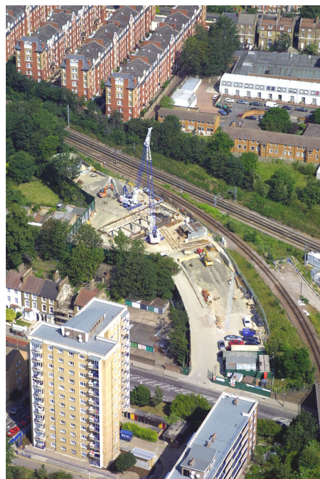
Fig. 6. Aerial photograph taken during shaft excavation showing the site's confined nature and residential surroundings.
