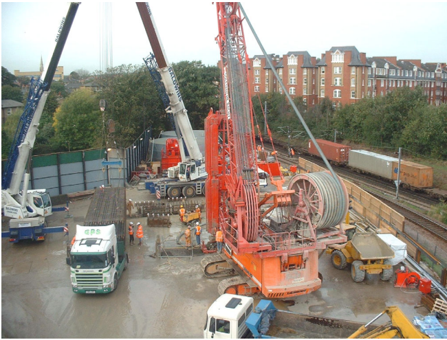
Fig. 4. Photograph showing delivery and lifting of a reinforcement cage section. The Bachy Soletanche Hydrofraise is seen in the foreground.
