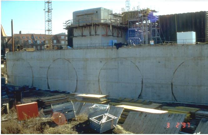
Fig. 5: Caisson used as starting pit for shield driven tunnels
