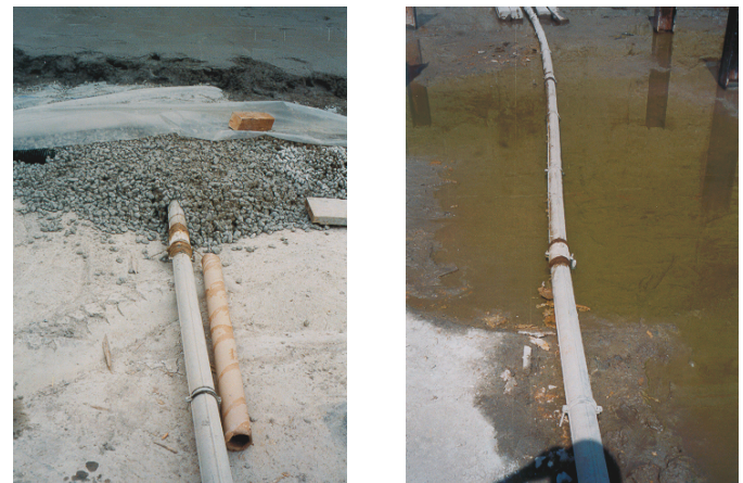
Fig. 9: Horizontal inclinometer for uplift measurement
