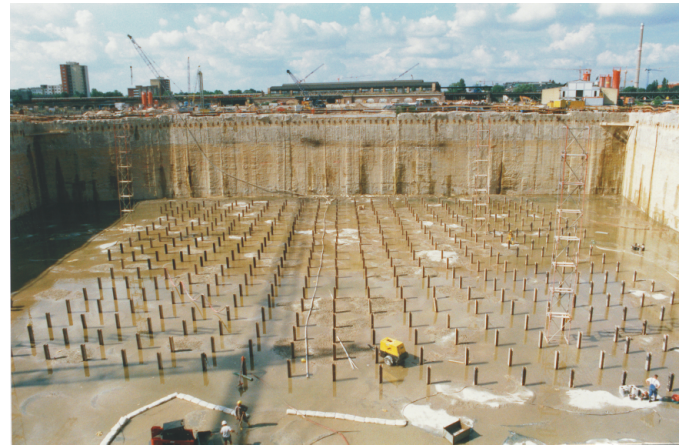
Fig. 8: Trough-type excavation after dewatering
