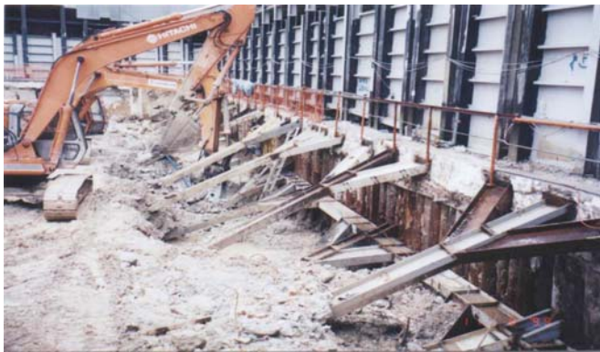
Plate 1 : Existing Basement Trimming Works
