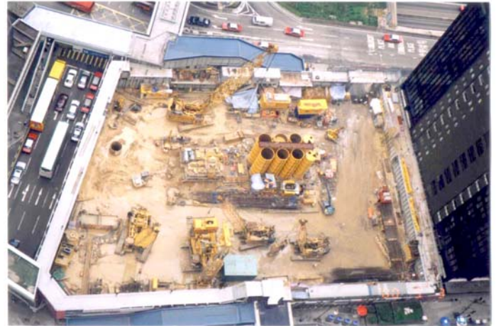
Plate 2 : Aerial View of Foundation Construction
