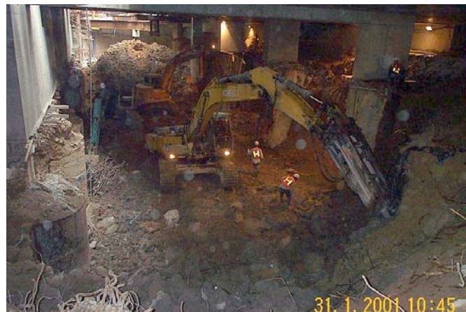
Plate 3 : Basement Excavation
