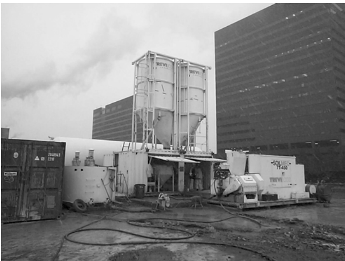
Fig. 10. Soilmec Soil Mixing Plant
