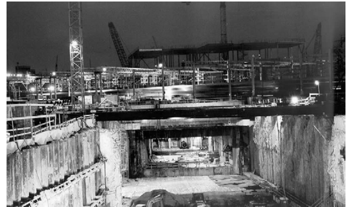
Fig. 11. Completed West Bound Tunnel Jacking Pit
