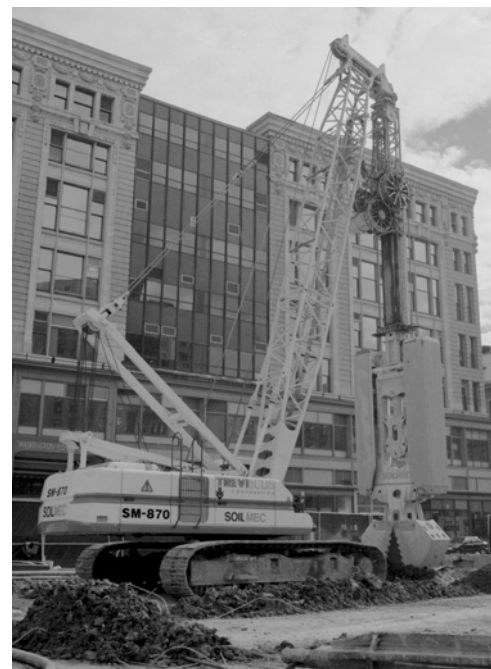
Fig. 8. Soilmec SM-870 with a BH-12 Hydraulic Clamshell
