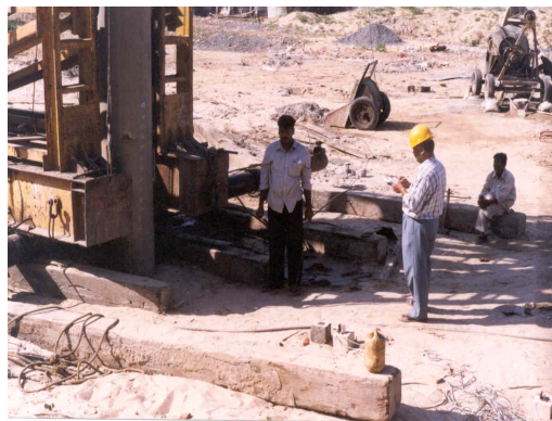
Partly driven pile
