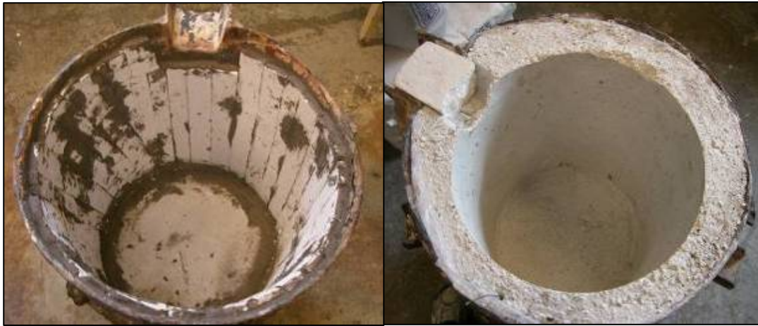
Figure 11. a) Insulation lining inside the steel shell b) ladle with cast commercial lining.
