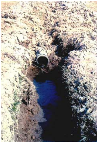
Slide 8. Outcoming water from geodrains
