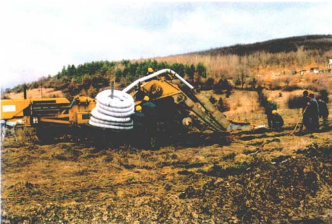
Slide 7. Construction of geodrains
