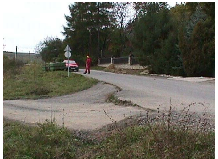
Slide 3. Transverse crack by the top of sliding surface
