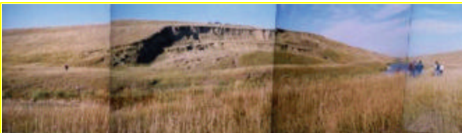
Fig. 5. Recent Slide on Right Side of Reach 2A Near Station 1160+00.
