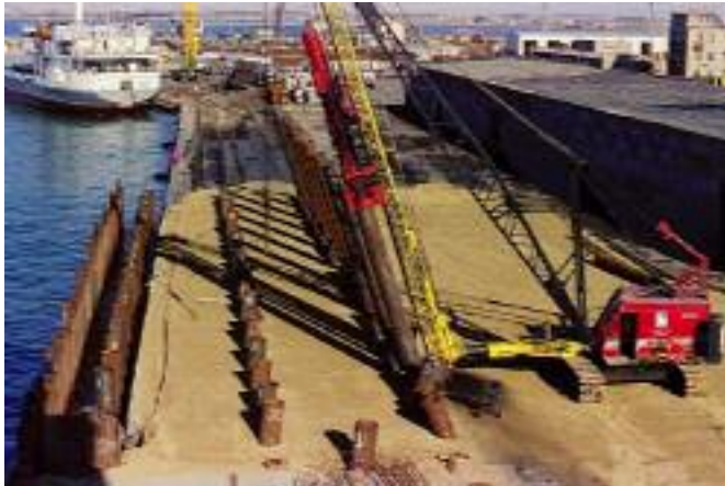
Fig 4. Installation of Raked Piles
