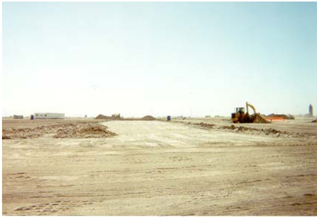
Fig. 5. Completed Foundation Pad for Cooling Tower Foundation Using Spoil Material.
