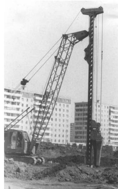
Fig. 2. General view of the unit and the tamper for the FTH construction on the site in the city Chelyabinsk
