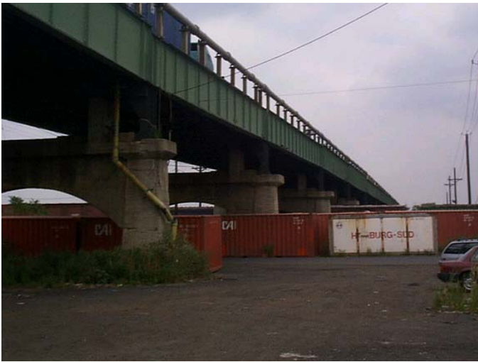
Fig. 1. The Old Doremus Avenue Bridge
