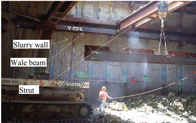
Fig. 1. SPTC wall braced by struts and walers
