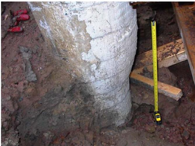
*Fig. 5. Necked pile showing a reduction in diameter of approximately 100mm, at Site B in Essex. Note: soil is very silty organic clay.*
