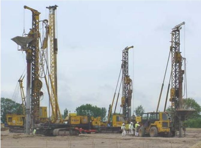
Fig. 13. Three stone column rigs undertaking ground improvement (foreground) and DCIS piling rig installing piles in ACC area (background left).
