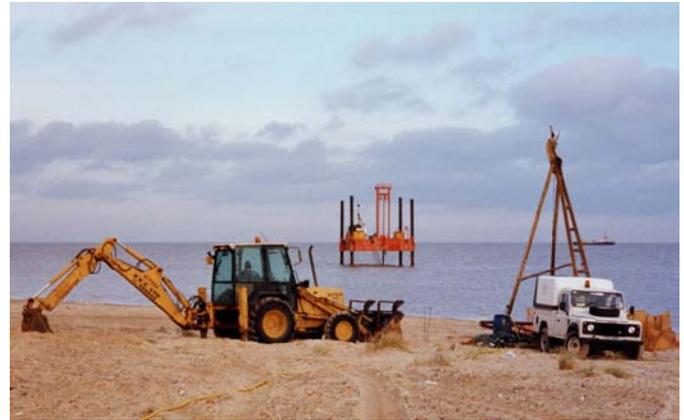
*Fig. 7. Onshore and offshore site investigation at Site C on the Norfolk Coast*
