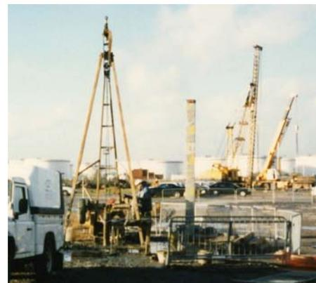
Fig. 4. Site investigation adjacent to a driven pile (foreground) with DCIS Piling (background) during piling trial.
