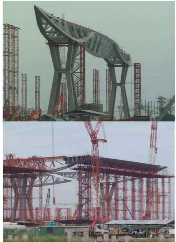
Fig. 9. Construction of typical Trellis Roof pylons (Super Columns) and Super Truss
