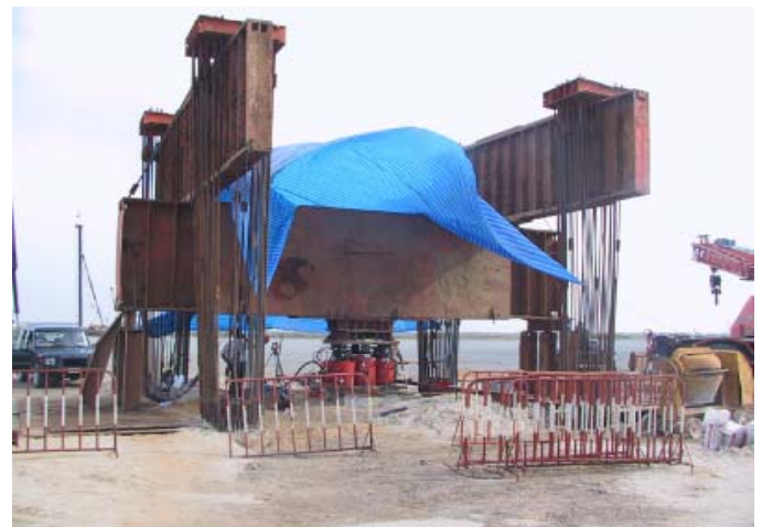
Fig. 7. Typical load test setup for a 1000 mm diameter bored pile
