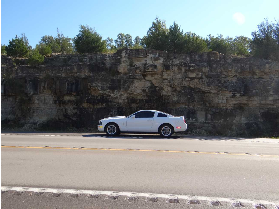
Figure 3: Site 2. Note the black stains on the rock indicating water flow.
