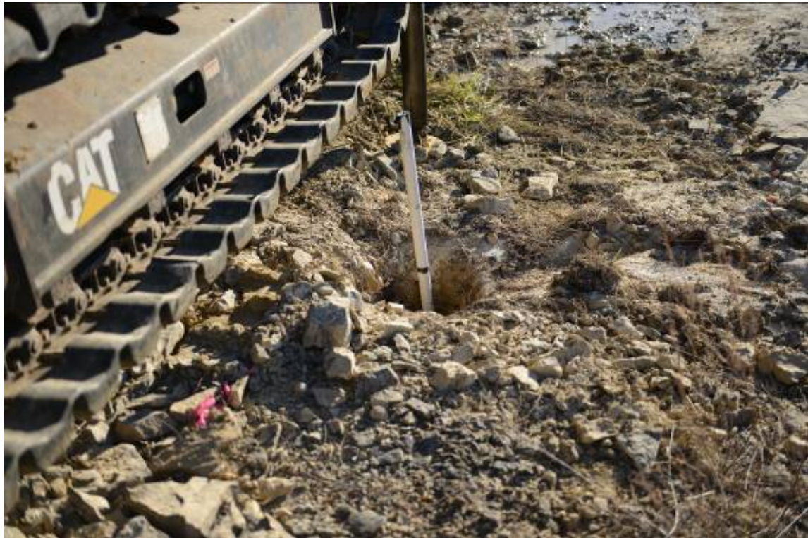
Figure 6: Piezometer installation.
