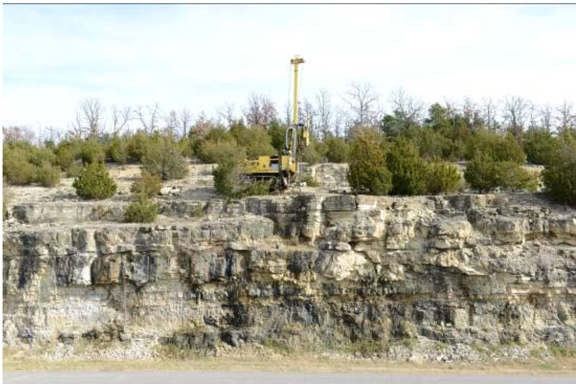
Figure 5: Core drilling on site 1.
