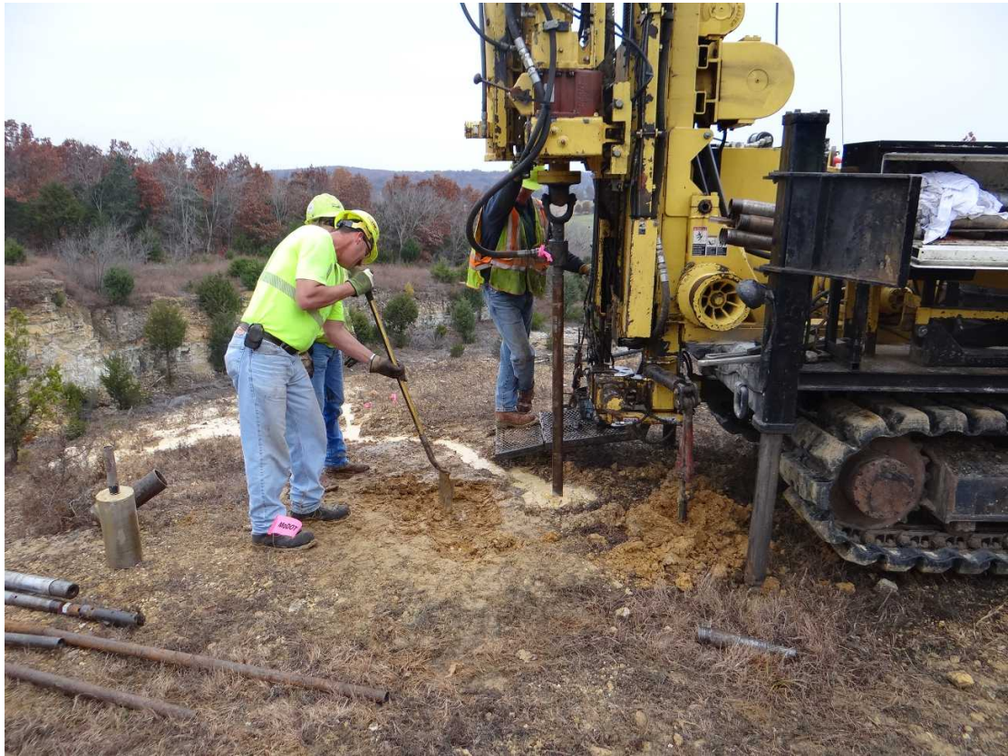
Figure 4: Core drilling on site 2.
