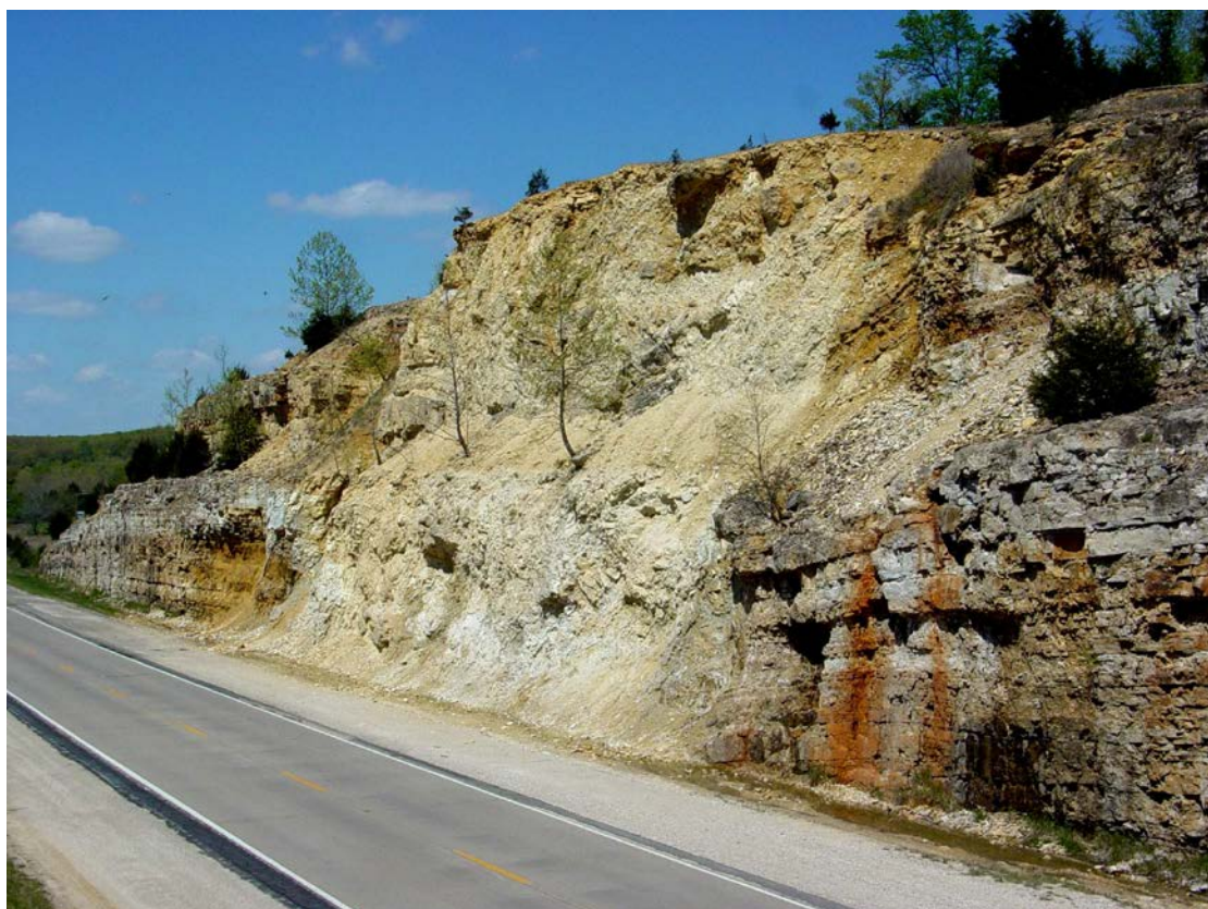
Figure 2: Site 1. This is a filled sinkhole that requires ongoing maintenance.
